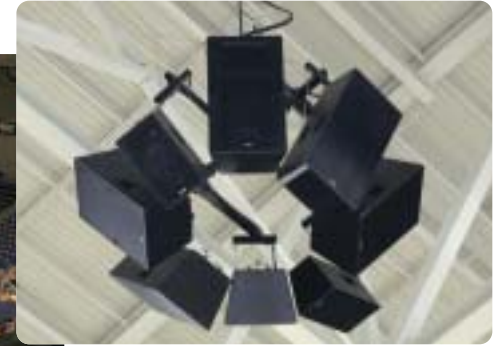
Gonzaga University's McCarthy Athletic Center features a center loudspeaker cluster, supported by end-court clusters, providing primary audio for the arena. The clusters consist of SLS series loudspeakers from Community (inset).
