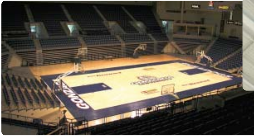
Gonzaga University's McCarthy Athletic Center features a center loudspeaker cluster, supported by end-court clusters, providing primary audio for the arena. The clusters consist of SLS series loudspeakers from Community (inset).
