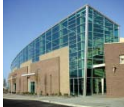
▲ Symetrix's SymNet takes control at Three Rivers Convention Center in Kennewick, WA.
